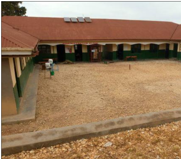
Before solar replacement
