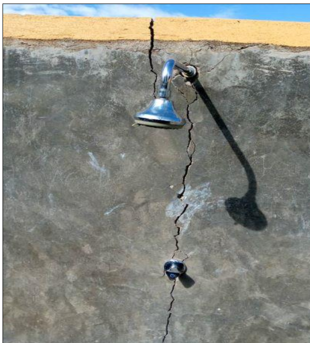
Crack before renovation
