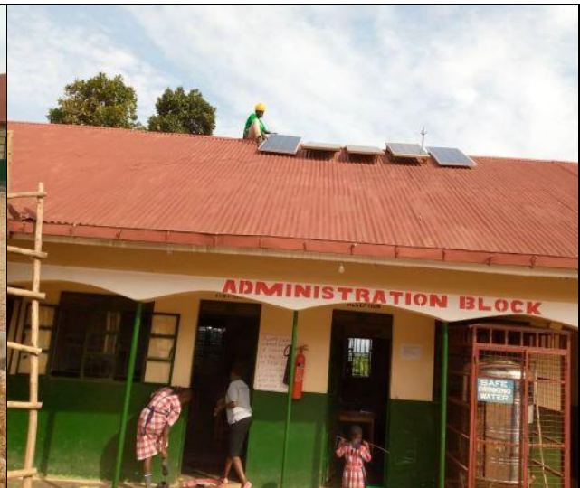
After replacing solar
