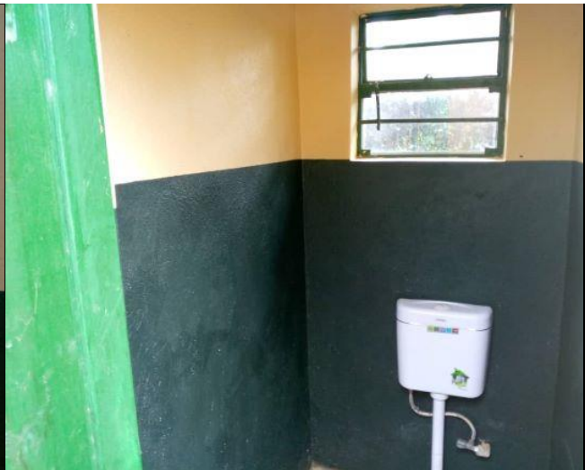
New paint in the girls' toilet
