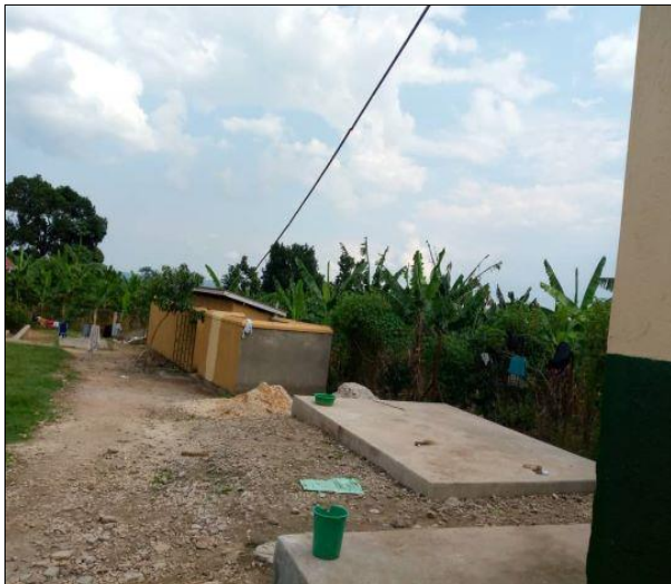
Electricity extension to the toilets
